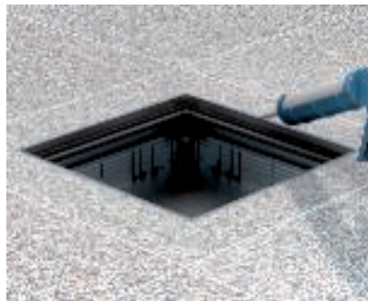
Laying the floor covering on the cassette frames RK/RKF Work the floor covering to the cassette frame. Seal the remaining gap between the floor covering and the cassette frame with suitable materials.
